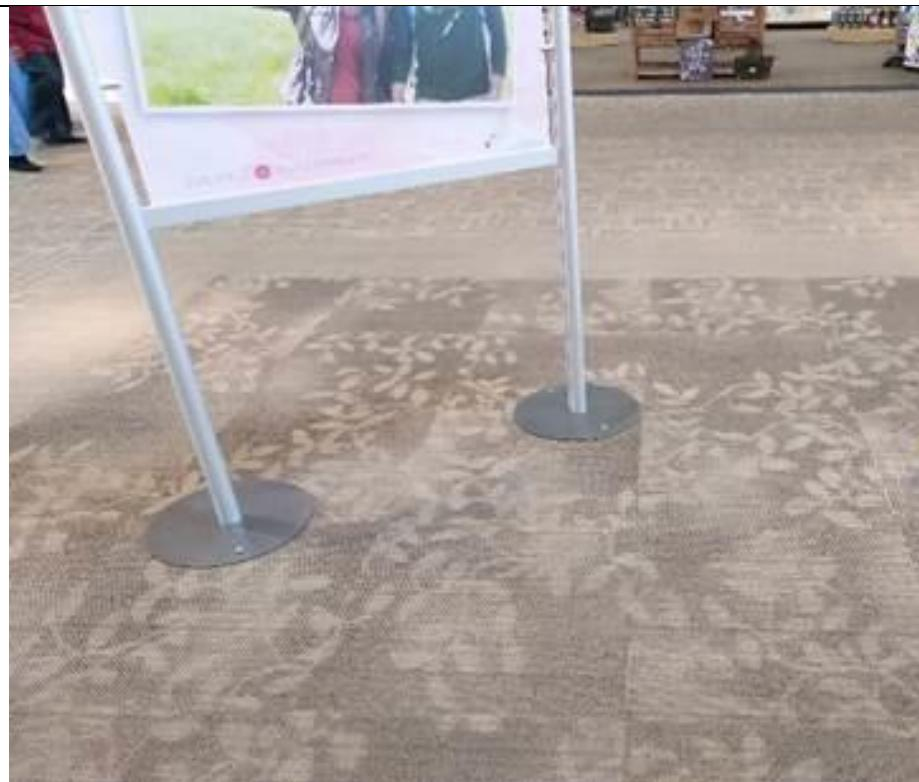
Each base will need to be secured with two bolts for a total of four per stand. Holes should be perpendicular to the bottom bar.
