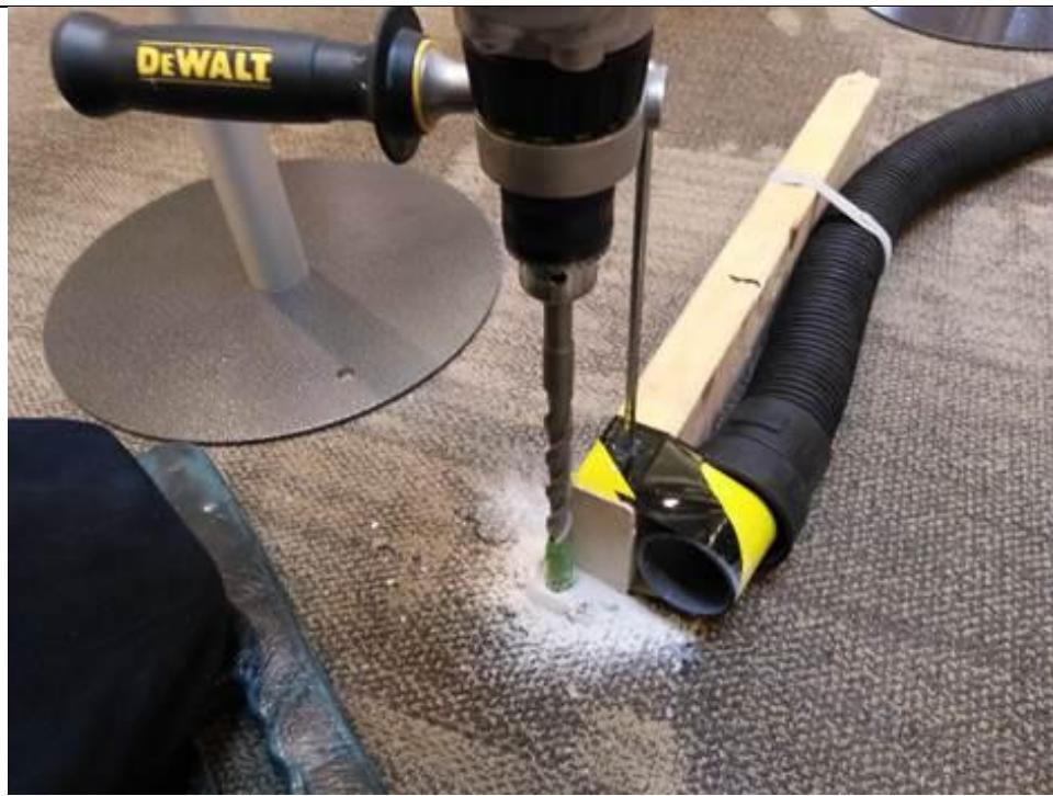
Set the stand aside then drill holes and slide in the lag shields. Vacuum system is optional.
