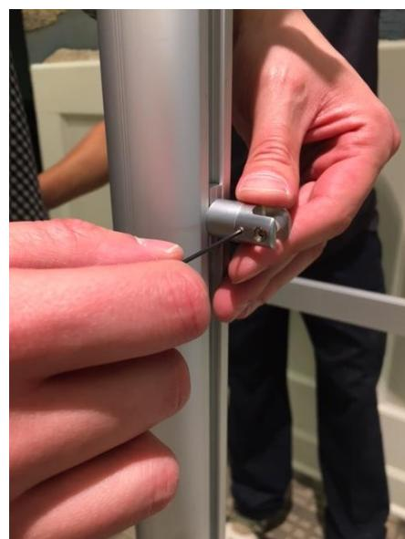
**Step 8:** Use the appropriately sized Allen wrench to open the standoff completely. The inside of the stand should appear completely open as shown below in the right photo below.
